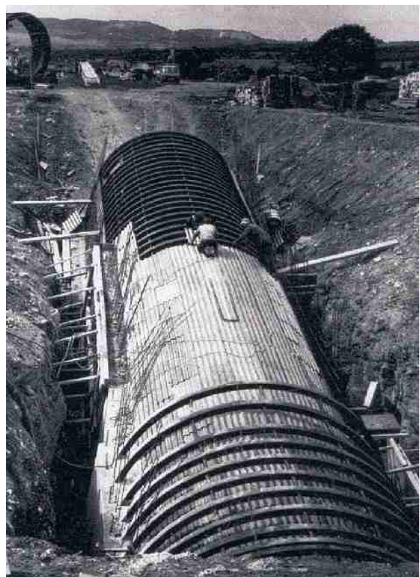
Image 4: Construction of Drift entrance June 1974
