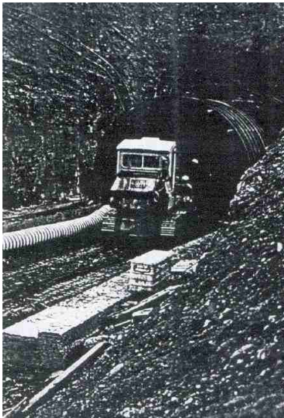
Image 3: Sinking the Drifts
