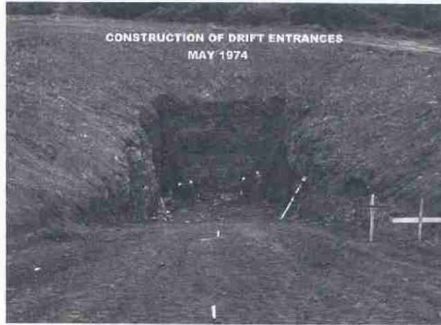
Image 2: Construction of Drift Entrance May 1974
