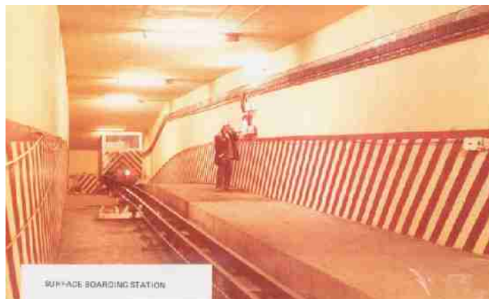
Image 8: Surface Boarding Station
