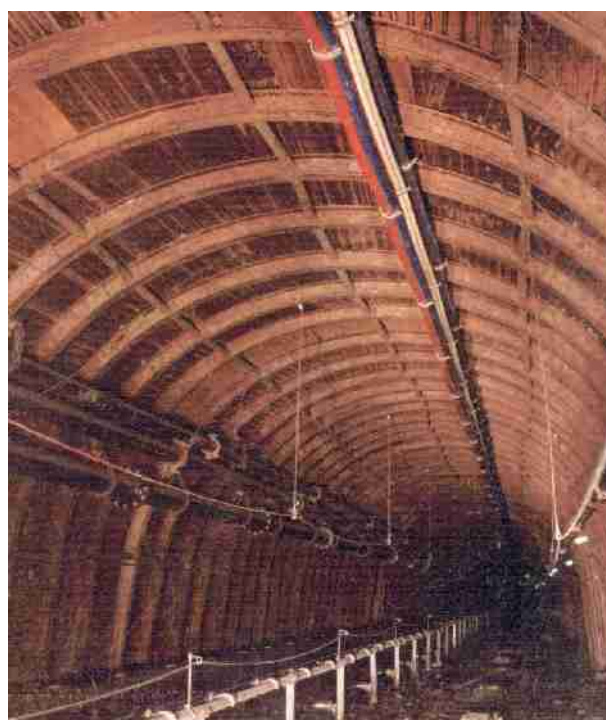
Image 11: Gate Road with a conveyor belt to carry the coal
